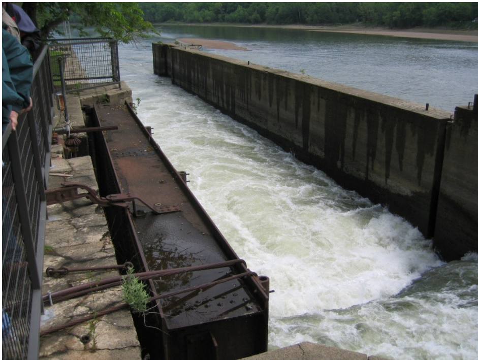
Lock chamber plunge pool and turbulence.
