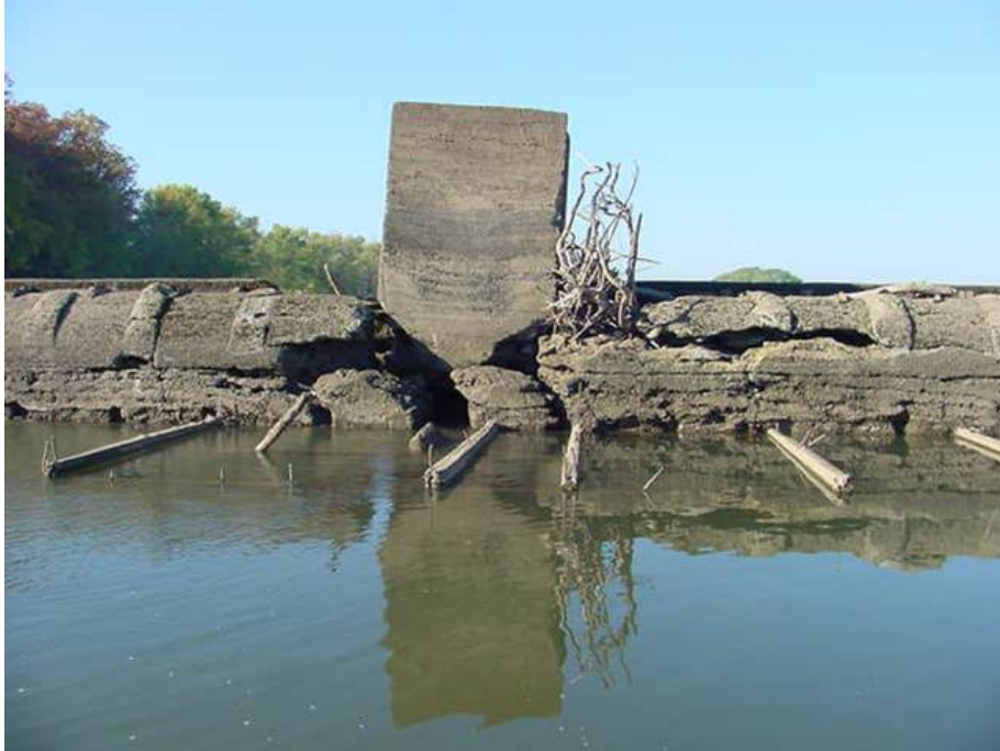
Photo credit: Bill Turner, Missouri Department of Conservation, 2005 Structural decay of L&D#1 dam sill and pillar.
