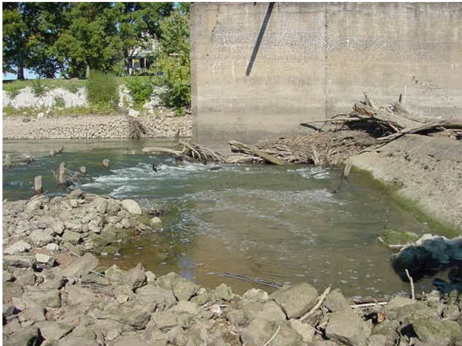
Whirlpool formed by undercutting of structure, upstream side of dam adjacent to lock wall.
