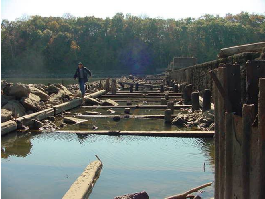
Photo credit: Bill Turner, Missouri Department of Conservation, 2005 Timber, steel and rock cribbing along downstream face of L&D#1.
