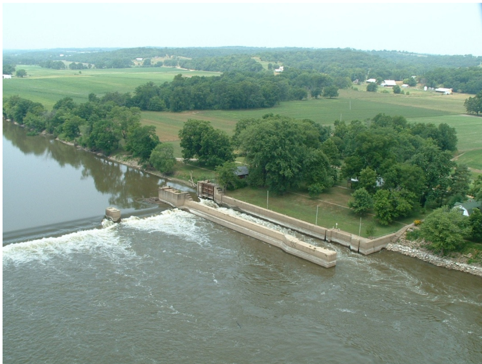
Aerial view of lock structure (center), sill and pillar of L&D#1.
