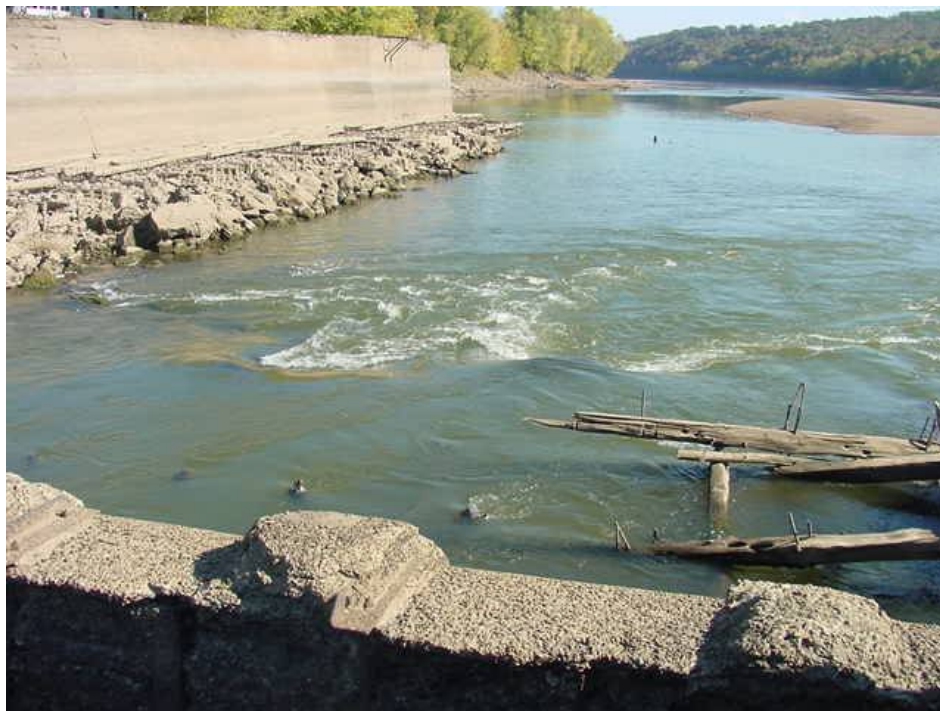
Photo credit: Bill Turner, Missouri Department of Conservation, 2005 Downstream flow from undercutting, adjacent to lock wall.
