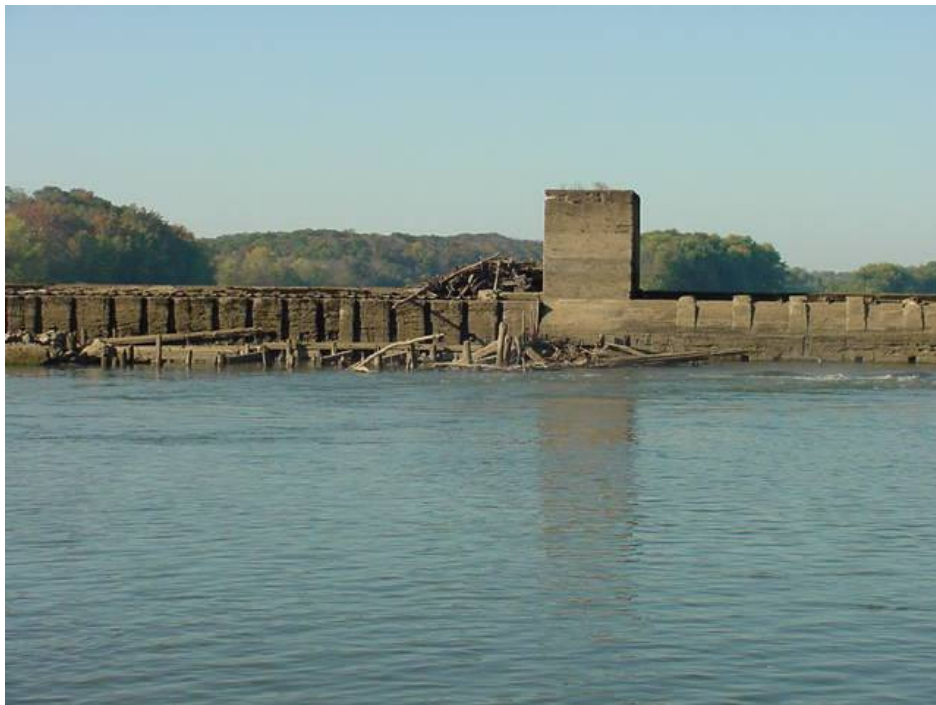
Downstream dam sill and pillar of L&D#1.
