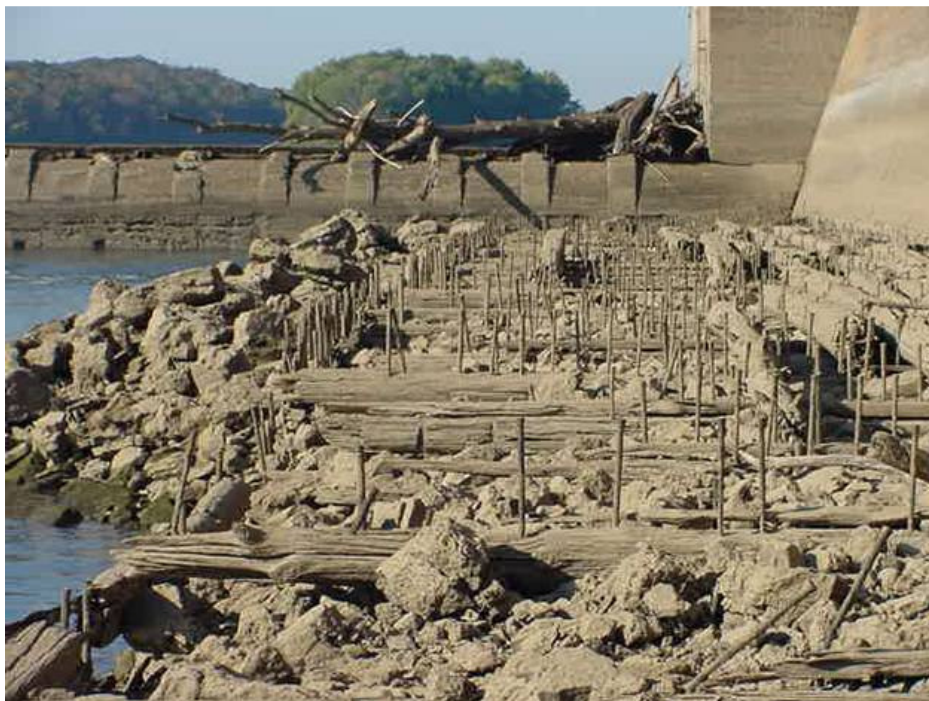
Photo credit: Bill Turner, Missouri Department of Conservation, 2005 Timber, steel and rock cribbing along lock wall (looking upstream, lock wall on right).
