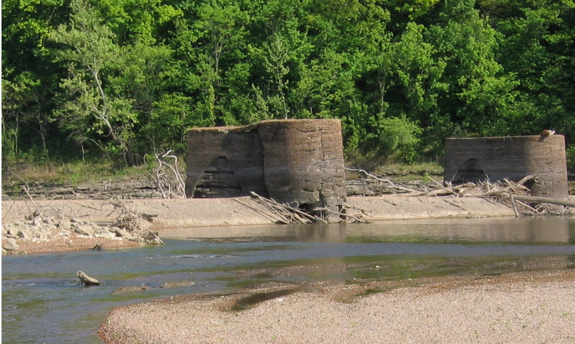
Upstream view of pillar degradation.
