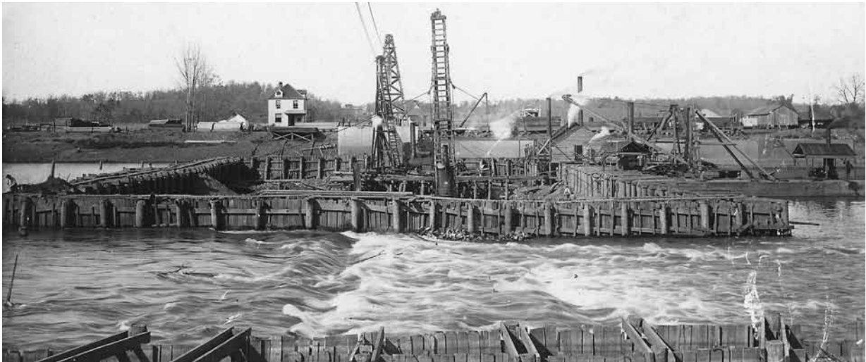
Above: Construction photograph of Lock and Dam No. 1.
